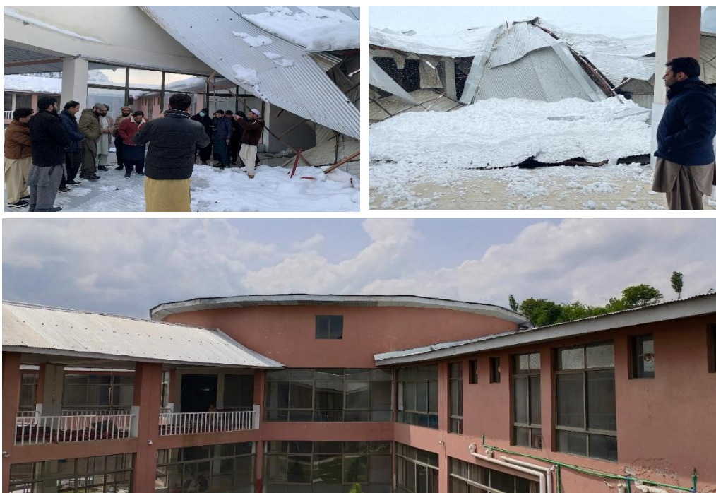
Dome fallen down due to heavy snowfall was repaired.
