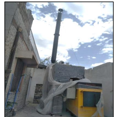
Newly installed incinerator
